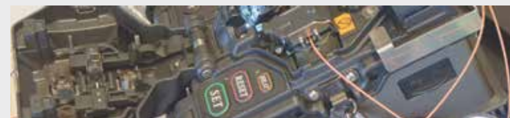
Welding, polishing and providing fiber optic cabling
